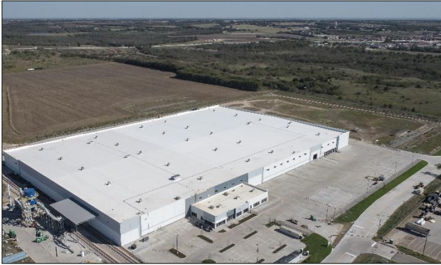
1. Entering the Hillsboro facility through the main road.
