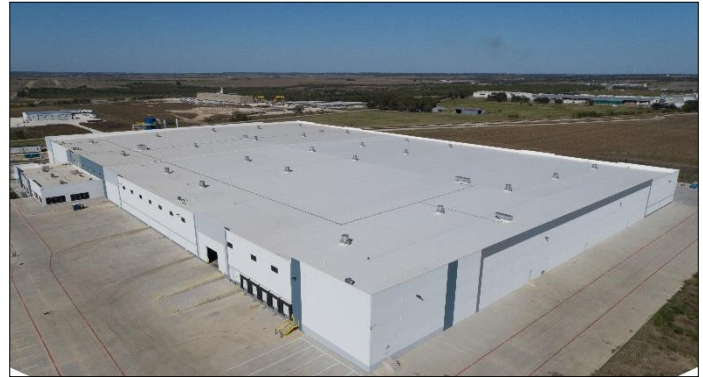
2. The distribution side of the Hillsboro facility.
