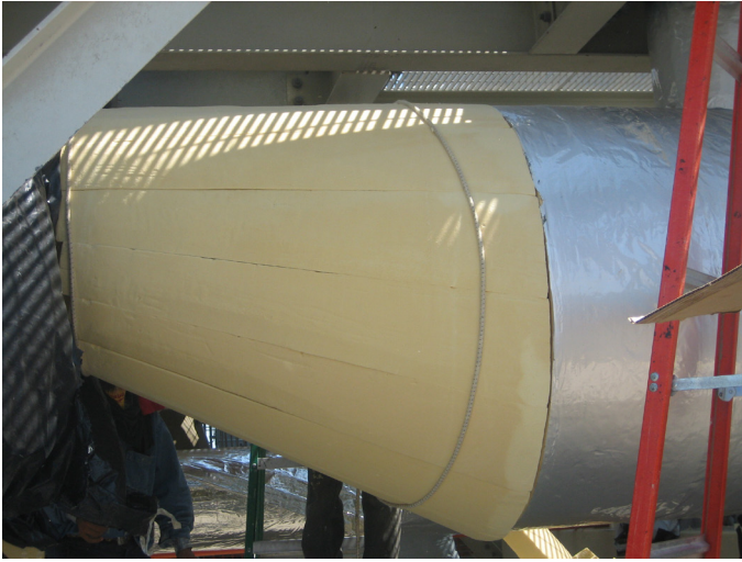
Figure 1. Trymer PIR is easily fabricated for a correct fit.
