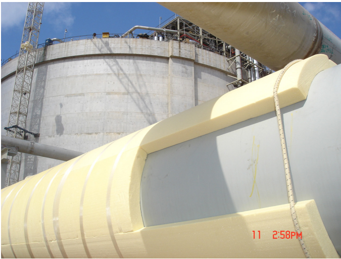
Figure 2. Trymer PIR offers lower total thickness.
